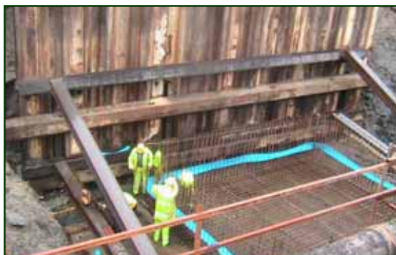
Castlebar Environs Sewerage Scheme – Construction of Sewage Pumping Station at Milebush
