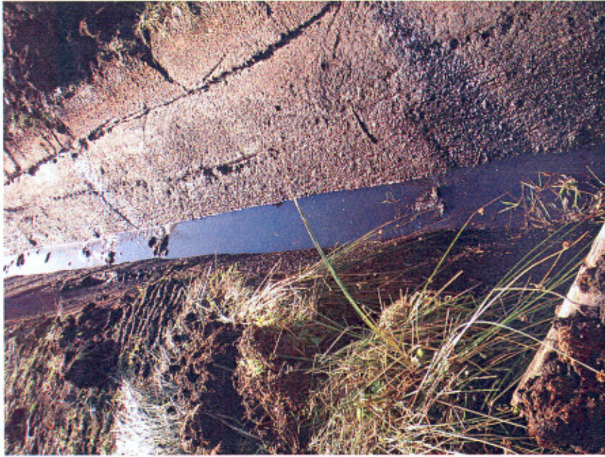
Figure No.3 View of Drain From Overtopping Area
