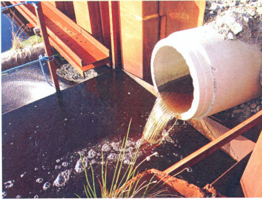
Figure No.5 View of Surfacewater Inflow To Settlement Ponds
