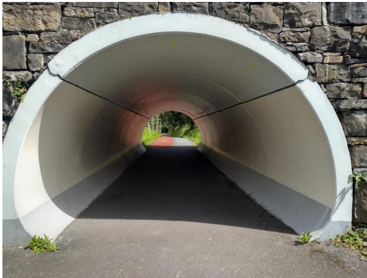
High street underpass 14 metres long 3.4 metres wide
