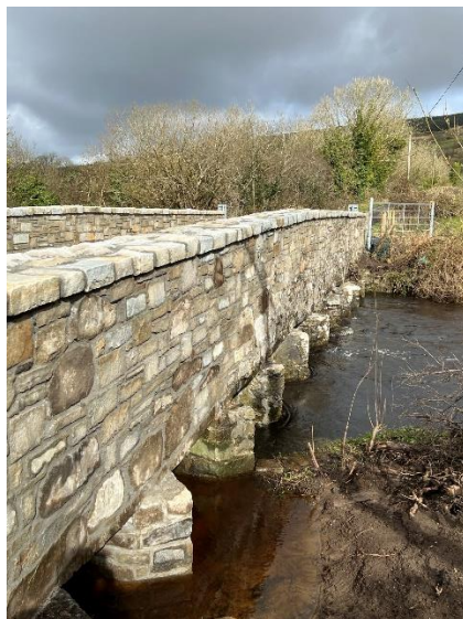
BRIDGE REHABILITATION WORKS AT KILKEERGLEN
