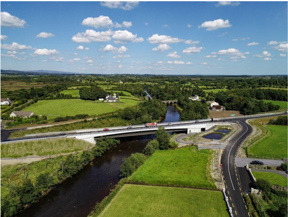
N26 REALIGNMENT AT CLOONGULLANE BRIDGE
