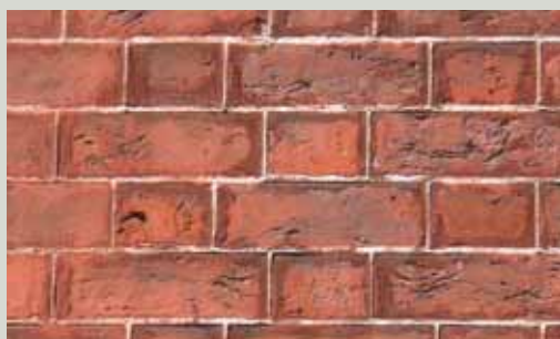
Façade with historic wiggled brickwork
