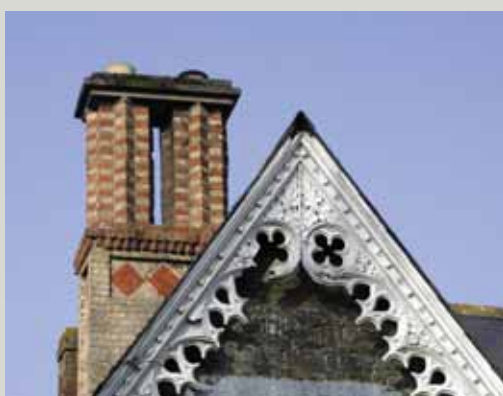
Decorative polychromatic brick chimneys at Castlebellingham, Co. Louth
