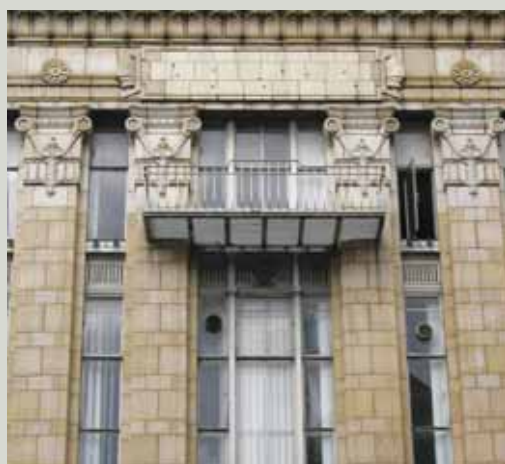
Burton's, Dame St, Dublin, designed in 1929 by Harry Wilson, is an example of high quality faïence cladding used to form a giant classical order to the façade
