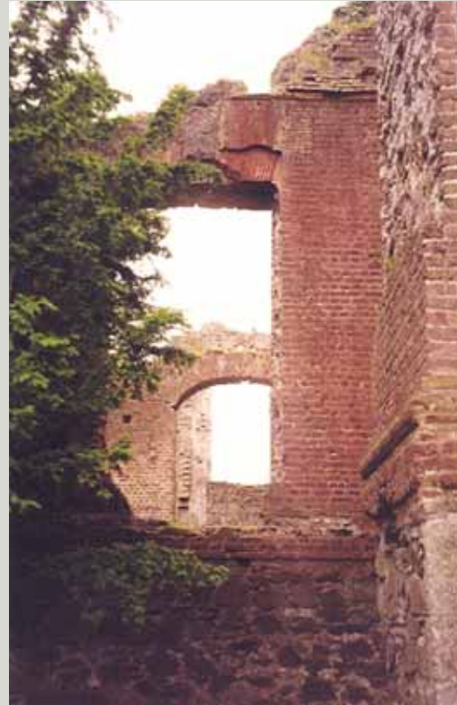
Jigginstown House, Naas, Co. Kildare, built c. 1637-40, is the first Irish building where imported brick and bricklaying expertise are believed to have been used although the majority of the bricks are thought to be of local origin
