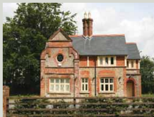
Groom's Cottage, Monasterevan, Co. Kildare, c.1882 constructed of machine-made red brick from Kingscourt, Co. Cavan and hand-made yellow brick from Athy, Co. Kildare
