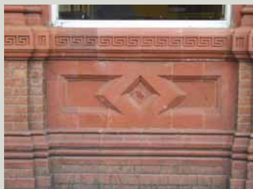
This terracotta panel has been carefully repaired following the removal of an automatic teller machine which had been inserted beneath the window
