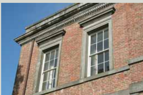
The brick façade, with stone dressings, of Cashel Palace, Co. Tipperary, was designed by Edward Lovett Pearce before 1729 for Archbishop Goodwin
