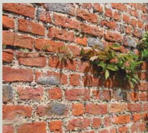
Garden walls lined with brick at Beaulieu House, Co. Louth. The orientation of garden walls was the subject of several gardening manuals in the early eighteenth century. The recommendations were that walls should face south-east, south-west, north-east and north-west. The first two, for example, were considered good for best fruit; the latter for plums, cherries and baking pears
