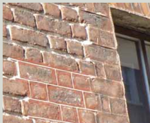
iii) the finished wiggging sample
