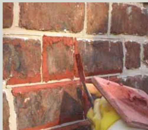
ii) laying in the pigmented stopping mortar up to the ribbon
