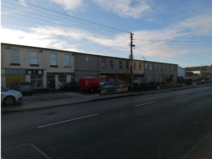
Photo 4.2 – Opportunity Site 1 (Hat Factory)
