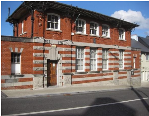
Photo 4.1: Redevelopment of the Former Castlebar Post Office to serve as a Community Youth Support Centre
