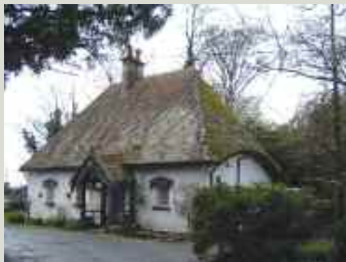
A gate lodge with a decorative clay-tiled roof, having striking curved elliptical eaves and a patterned use of plain and scalloped tiles. Overhanging branches and the proximity of large trees have tended to promote extensive moss growth on part of the roof
