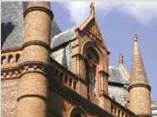
Victorian roofs are often architecturally complex, using a variety of roof shapes, roofing materials and embellishments
