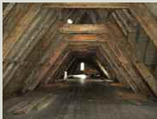
A late sixteenth-century oak roof over a large hall at Ormond Castle, County Tipperary
