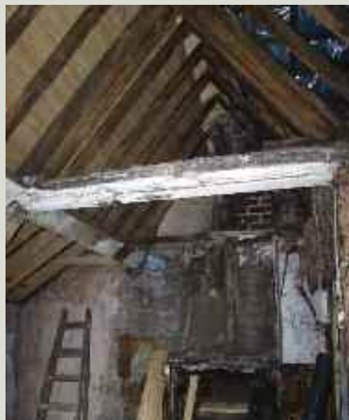
An early-seventeenth century roof showing the original principal roof structure and rafters with replacement sarking boards above (Image courtesy of Tom McGimsey, Mesh Architects)
