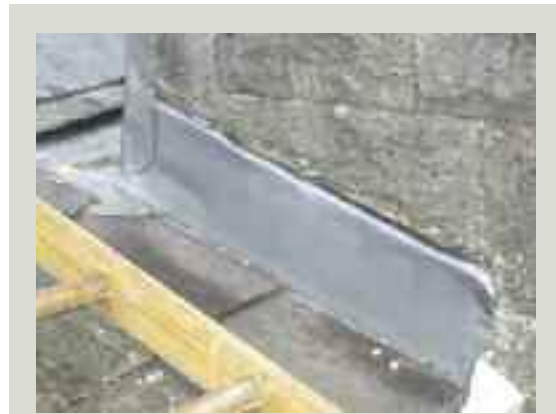
New lead flashing over lead soakers, turned into a mortar joint in the stonework at the base of a chimneystack and fixed using lead welts. The mortar joint is yet to be repointed
