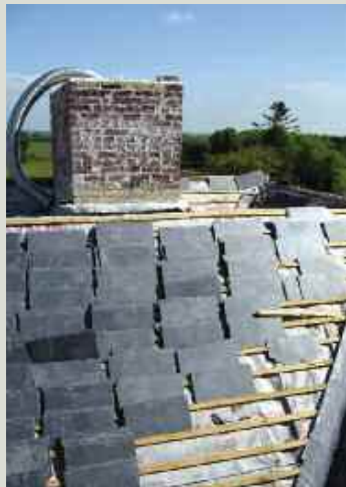
Flexible stainless steel flue being inserted into a historic masonry flue
