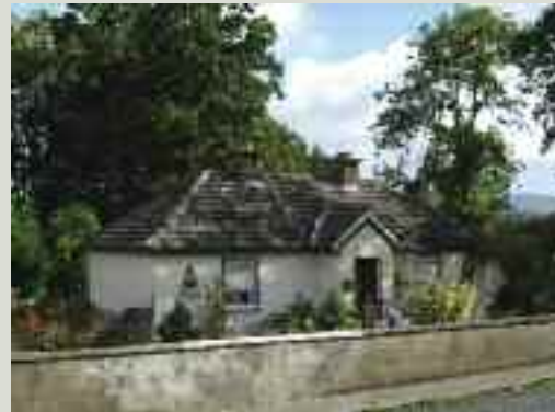
A Marley concrete roof tile on this modest 1940s cottage
