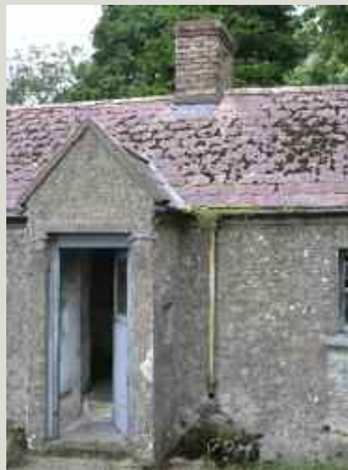
Asphalt shingles were introduced as early as 1890, although their use is more usually associated with buildings dating from the 1930s
