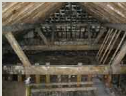
An eighteenth-century re-roofing of a tower house using imported deal
