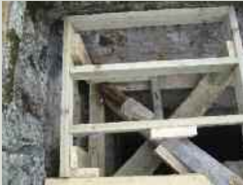
Additional support was added on the diagonal below the truss end, thus avoiding the need for new timber splice and steel connections or the local removal of the rotten timber truss end. The timber that had supported the gutter above had to be fully replaced
