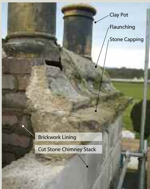
Chimneystacks were traditionally constructed of coursed brick or stone, gathering numerous flues into a single large masonry element often finished off with a stone capping
