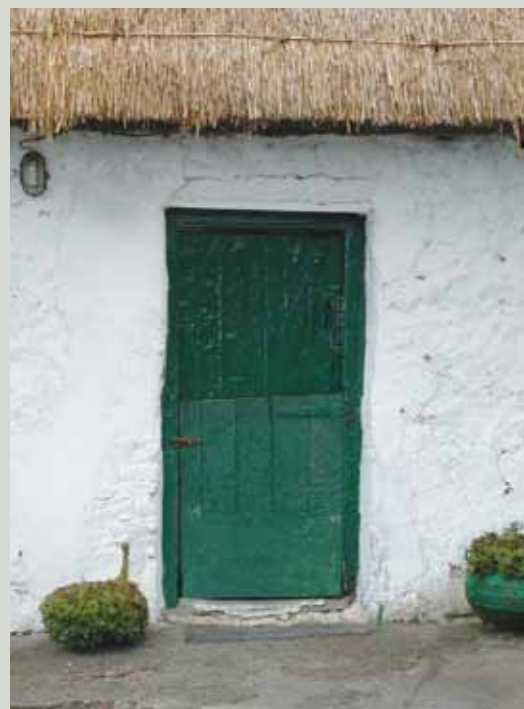
A traditional timber half door
