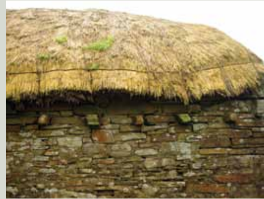
An example of roped thatch in County Donegal. Ropes passed over the roof at regular intervals secure the thatch against high winds and are tied to stones projecting from the walls
