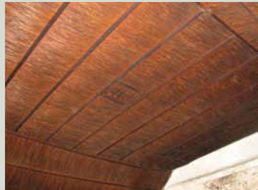
Ceiling made from reed fleeking
