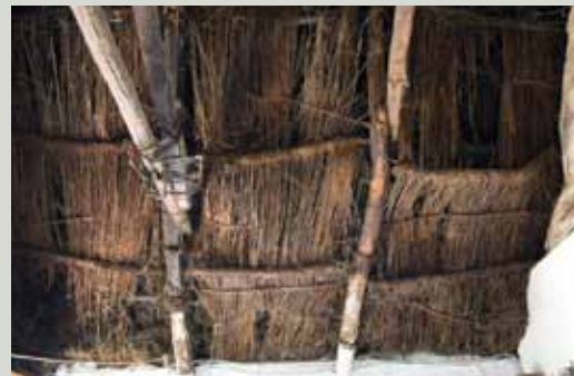
Straw lining to the underside of a roof in County Limerick
