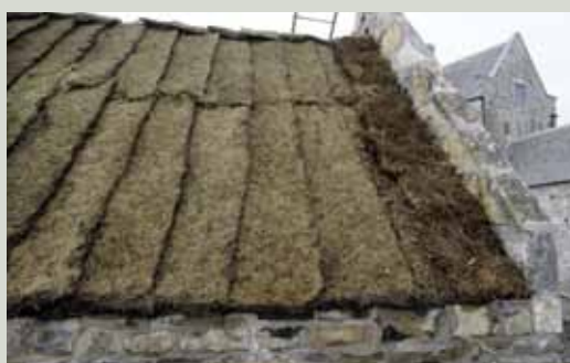
Scraw laid on a reconstructed roof
