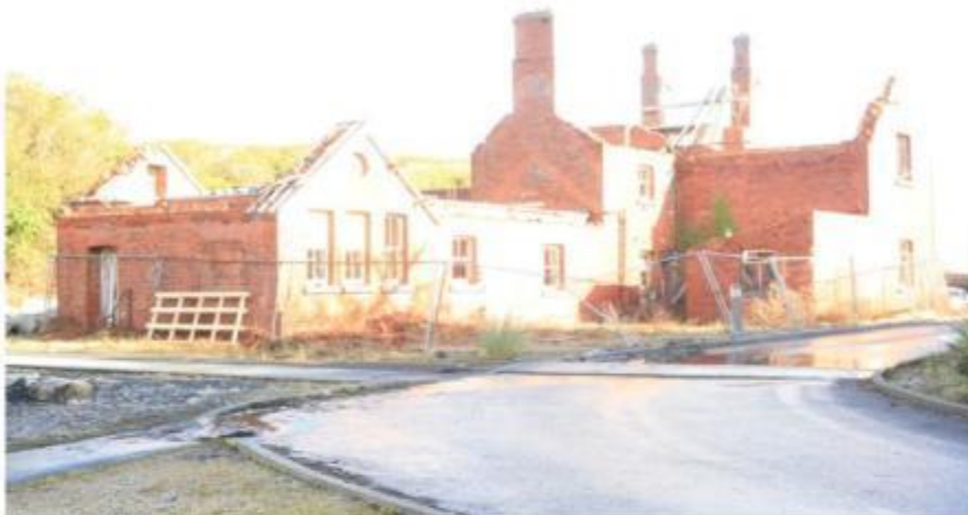
View to rear of building (facing N-E) prior to reconstruction works – February 2016
